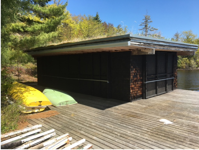
North West corner
